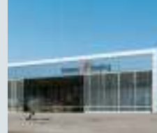
Ameco A380 Hangar Peking, China
