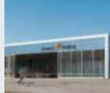
Ameco A380 Hangar Peking, China
