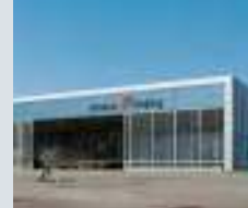
Ameco A380 Hangar Peking, China
